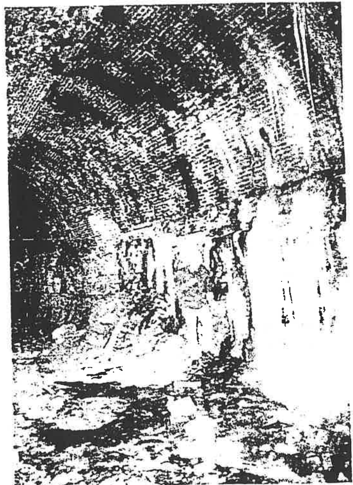
Photograph No. 11: Failure of Horizontal (Ceiling) Member of Timber Bent at Station 14+35±. Note Excessive Deflection on Fourth Bent from Top of Photograph
